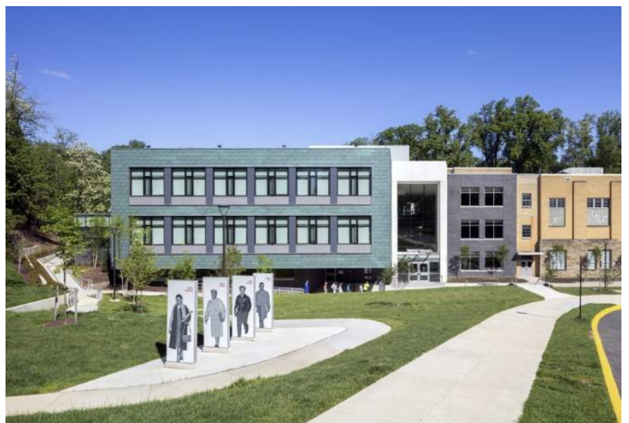
Figure 8 - Dorothy Hamm Middle School new main entrance. Image courtesy of Quinn Evans; photographer Joe Romeo.
