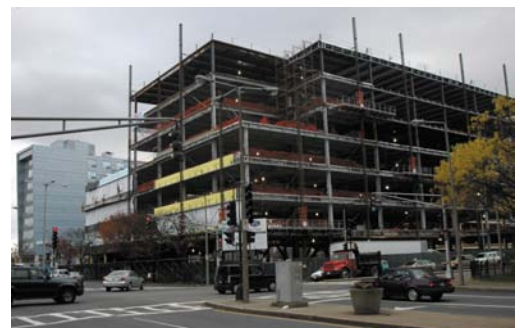
Crosstown Phase 2: Office Building
