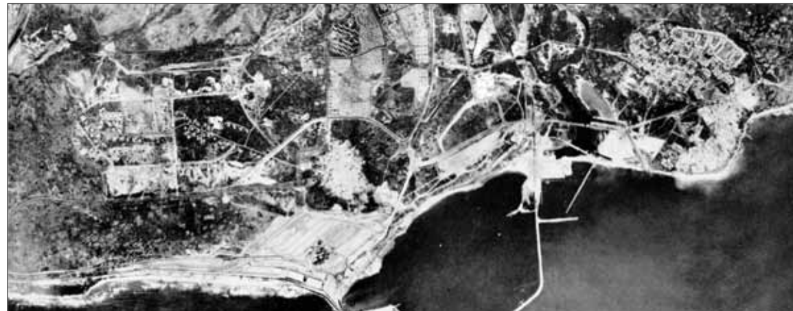
Aerial view of Tema under construction, November, 1959. Distance left-to-right is 3.5 miles.
